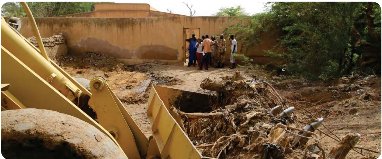
Douentza prison under rehabilitation
