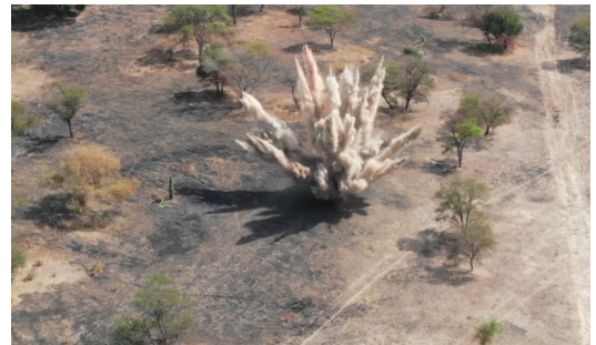
Demolition in Khar Alei
